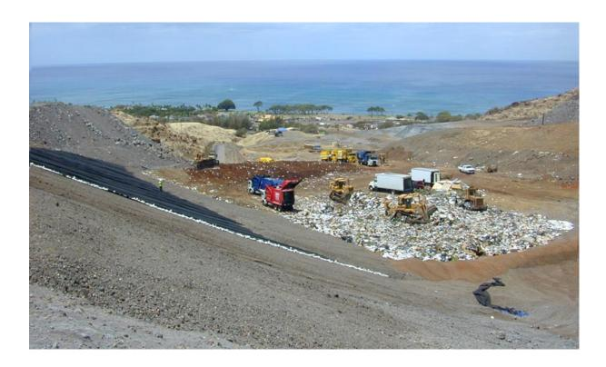
Figure 5.27: A landfill site in Hawaii, USA. The base of the old quarry and the sloping sides have been covered with a black plastic landfill liner (membrane) to ensure that fluids don't leak into the surrounding rock; this is then covered by gravel for protection.
