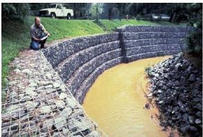
Figure 6.13: Stone-filled gabions, stabilising a river bank.
