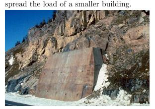
Figure 6.12: A retaining wall supporting weaker materials in a cutting.
