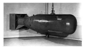
Figure 16.2: A replica of the nuclear bomb dropped on Hiroshima. This was a gun-type bomb, where two subcritical masses of highly enriched uranium were rapidly driven together by means of conventional explosives.
