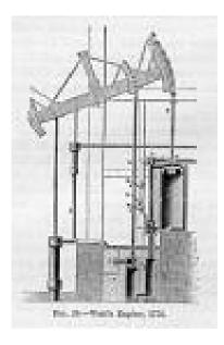
Figure 8.4: One of Watt's engines. These engines supplied the power needed for factories, mines and transportation during the Industrial Revolution.
