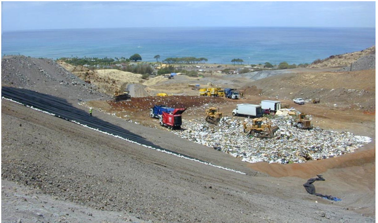
Figure 5.27: A landfill site in Hawaii, USA. The base of the old quarry and the sloping sides have been covered with a black plastic landfill liner (membrane) to ensure that fluids don't leak into the surrounding rock; this is then covered by gravel for protection.
